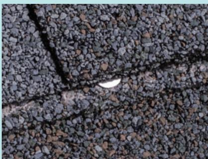
Some nailing lines are set close to the shim. This can leave nail heads exposed after installation, which creates unsightly 'shiners' that reflect light and detract from the beauty of the roof.
