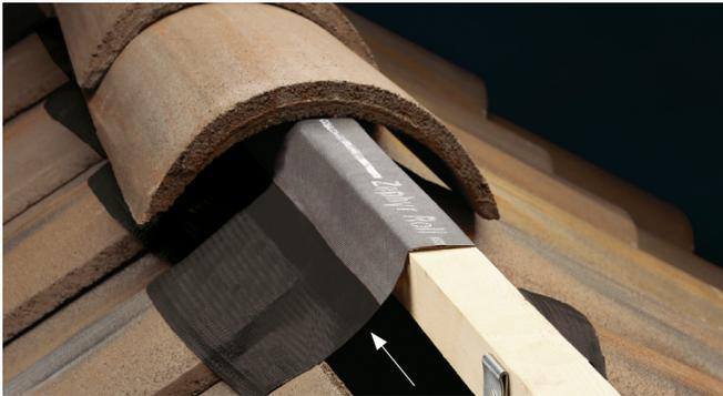
**NOTE: Ensure there is no low point after installation that would allow water to collect.**
