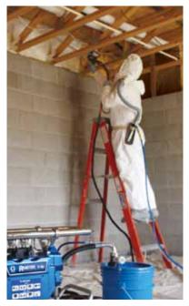
The Reactor E-8p is the best choice for portability and high-quality spray foam since it's lightweight and compact at 95 pounds, and can be plugged into one 115V outlet.
